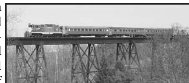
Crossing the River Styx trestle, spring of 2013. (Richard Jacobs)
